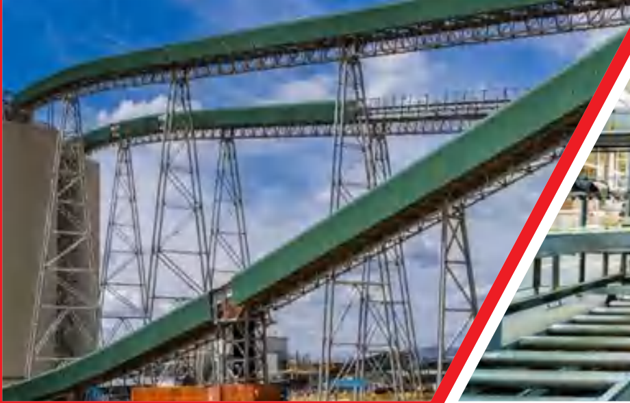
MADEN TESİSİ MINING PLANT
